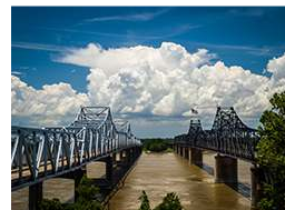
I-20 and Old Highway 80 Bridges
