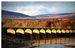
Dividing Weir Bridge
