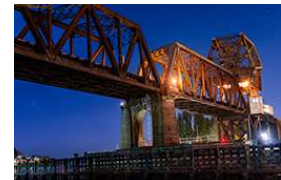
Salmon Bay Bridge
