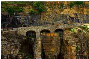
Triple Arches Bridge
