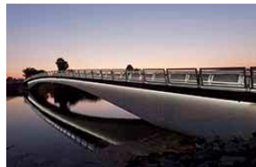
Mike Gotch Memorial Bridge
