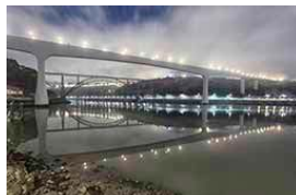
St. John's Bridge
