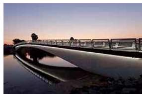
Mike Gotch Memorial Bridge
