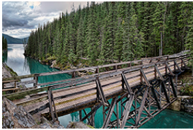
Stewart Canyon Bridge
