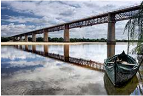
Dom Luis Bridge
