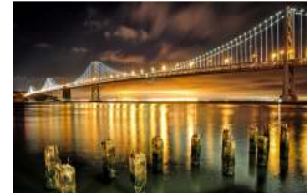
SF-Oakland Bay Bridge
