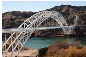
Old Trail Rt. 66 Bridge
