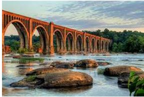
ACL Railroad Bridge
